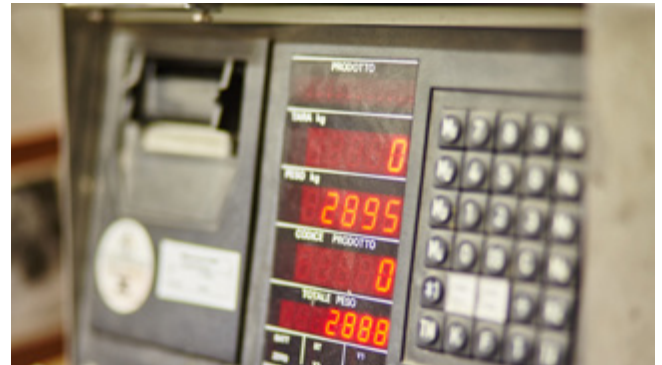
Electronic weighing of 100% of vehicles before delivery and written weight certification for end customer.
