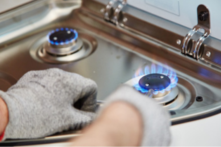
Test on operation of the gas pipes.
